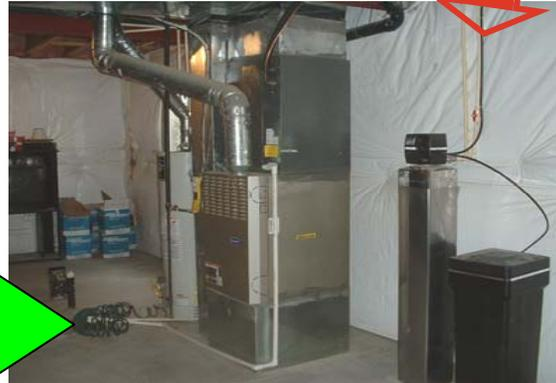
District Staff has observed cases of improper installation of water softeners that have resulted in direct cross-connection between water and sewer lines.
